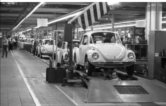
Asamblarea Volkswagen Beetle la Wolfsburg, Germania (anii '60)
